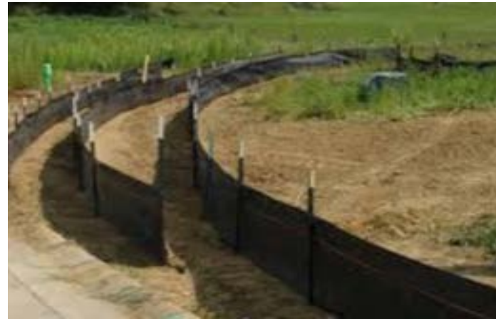
Figure 9: Proper placement of silt fencing for slopes
